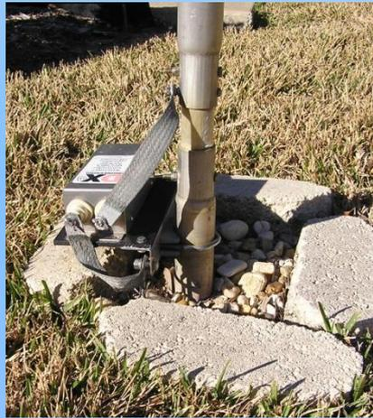
Pipe Support with Isolated Core Rod
