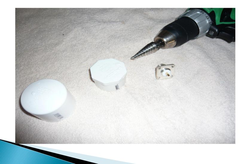
Insert the connector into the hole ,connection side out, the and mark and drill 2 holes for the support screws and nuts.
