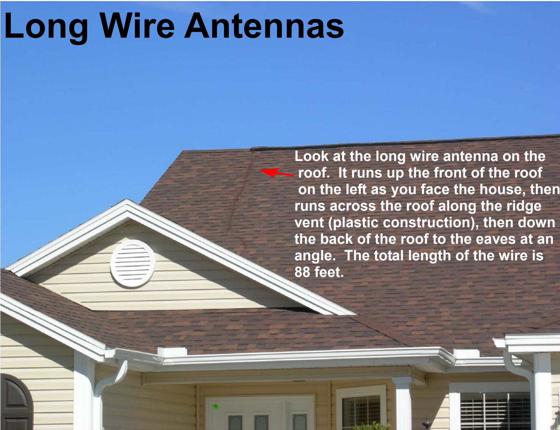
Look at the long wire antenna on the roof. It runs up the front of the roof on the left as you face the house, then runs across the roof along the ridge vent (plastic construction), then down the back of the roof to the eaves at an angle. The total length of the wire is 88 feet.
