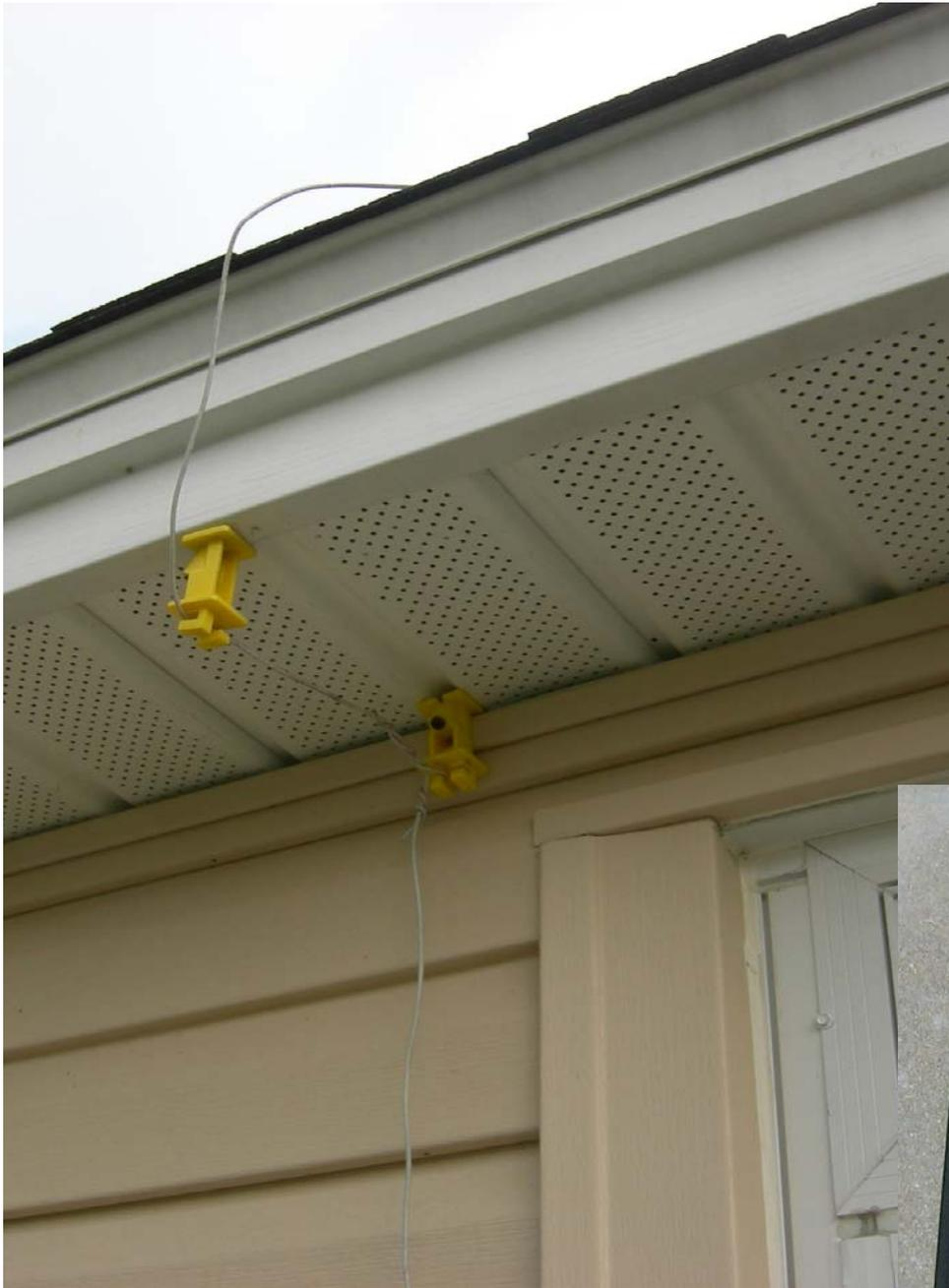
The wire from the roof drapes over the eave to an electric fence insulator seen here as yellow, then it goes down the side of the house to a hole in the siding where it enters the house shown on the next page. Elsewhere, he uses electric fence insulators, as shown above, easily obtainable at farm supply stores such as TSC, Menards, Lowe's, Home Depot, or Fleet Farm to secure the wire and hold it off the siding. (another idea to which we shall return).
