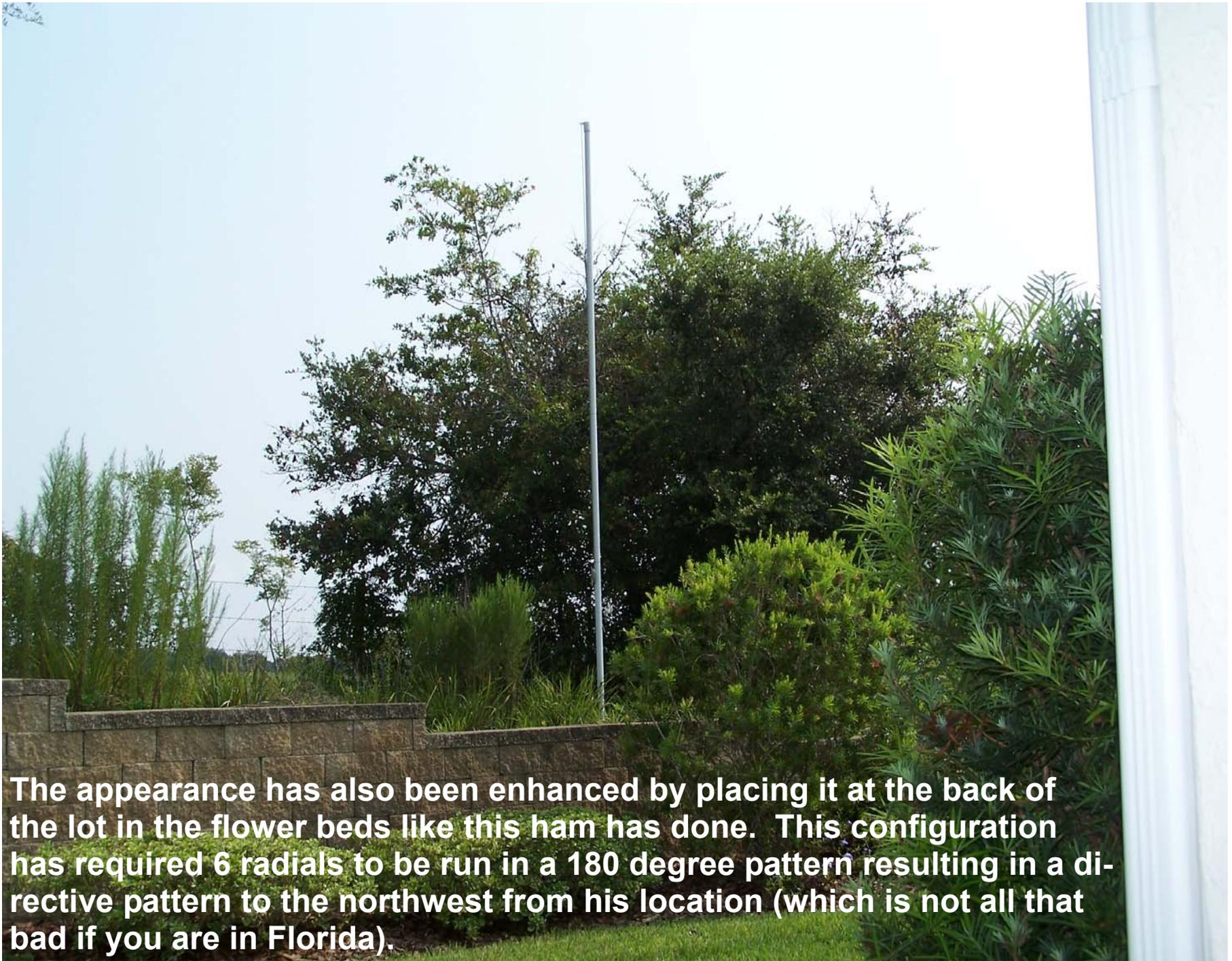
**The appearance has also been enhanced by placing it at the back of the lot in the flower beds like this ham has done. This configuration has required 6 radials to be run in a 180 degree pattern resulting in a directive pattern to the northwest from his location (which is not all that bad if you are in Florida).**
