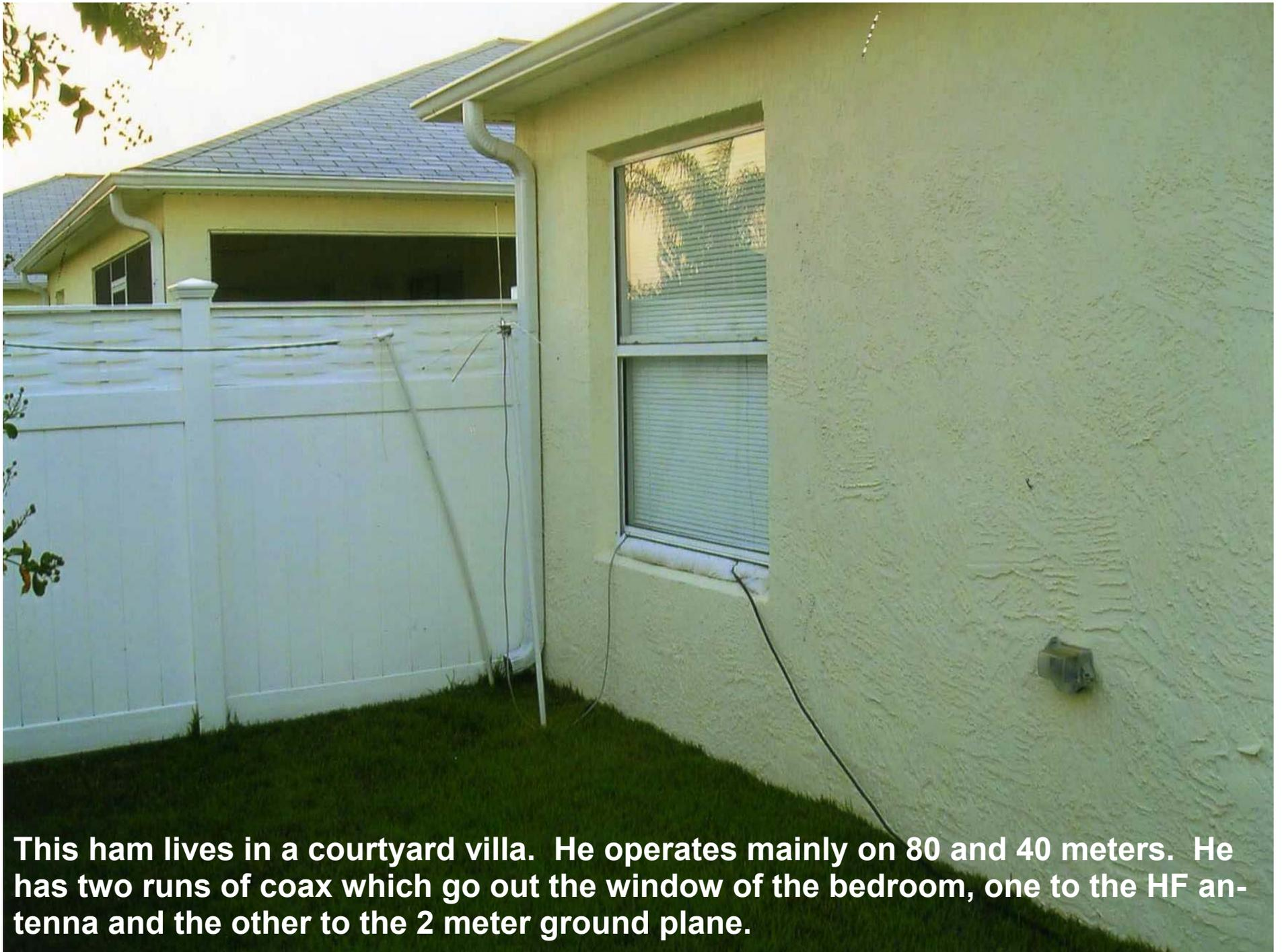
**This ham lives in a courtyard villa. He operates mainly on 80 and 40 meters. He has two runs of coax which go out the window of the bedroom, one to the HF antenna and the other to the 2 meter ground plane.**
