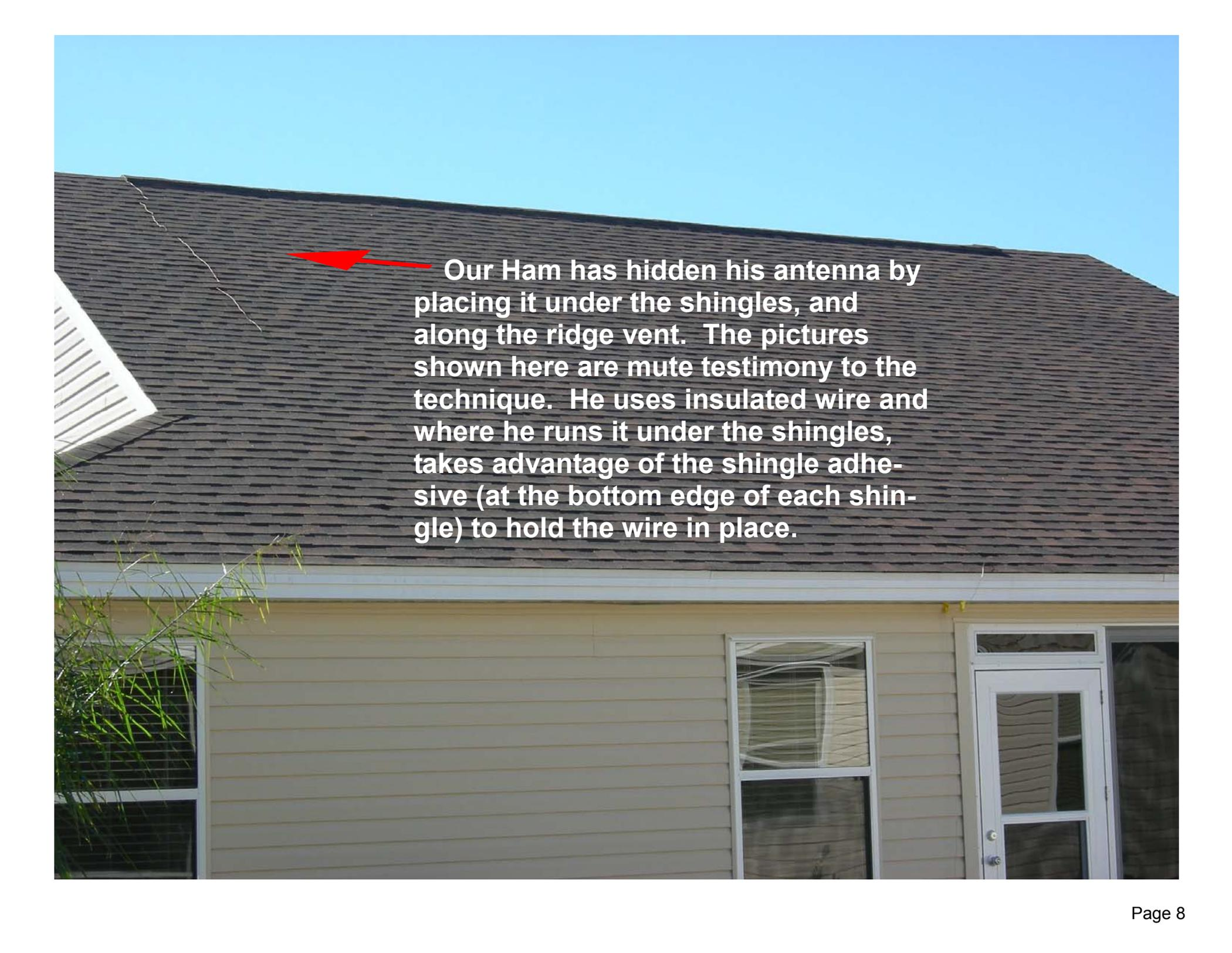
**Our Ham has hidden his antenna by placing it under the shingles, and along the ridge vent. The pictures shown here are mute testimony to the technique. He uses insulated wire and where he runs it under the shingles, takes advantage of the shingle adhesive (at the bottom edge of each shingle) to hold the wire in place.**
