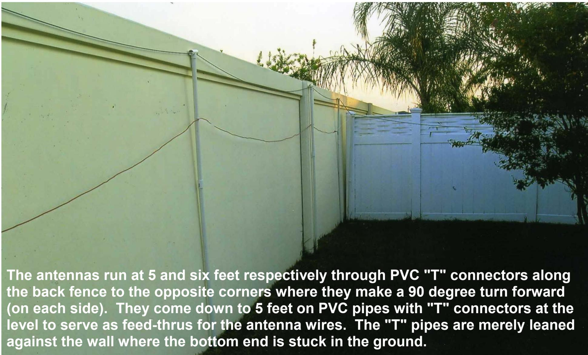
**The antennas run at 5 and six feet respectively through PVC "T" connectors along the back fence to the opposite corners where they make a 90 degree turn forward (on each side). They come down to 5 feet on PVC pipes with "T" connectors at the level to serve as feed-thrus for the antenna wires. The "T" pipes are merely leaned against the wall where the bottom end is stuck in the ground.**
