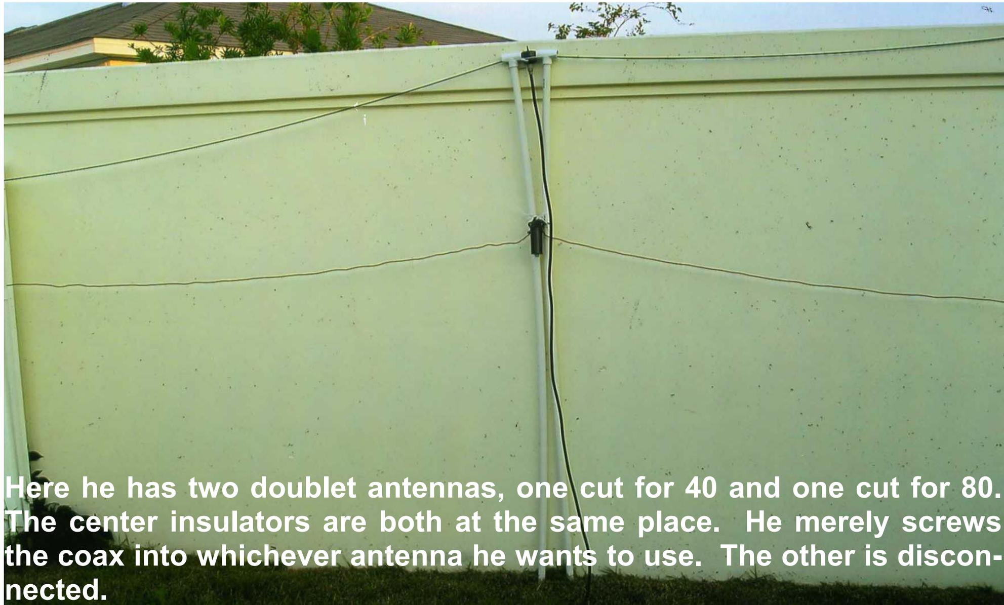
Here he has two doublet antennas, one cut for 40 and one cut for 80. The center insulators are both at the same place. He merely screws the coax into whichever antenna he wants to use. The other is disconnected.
